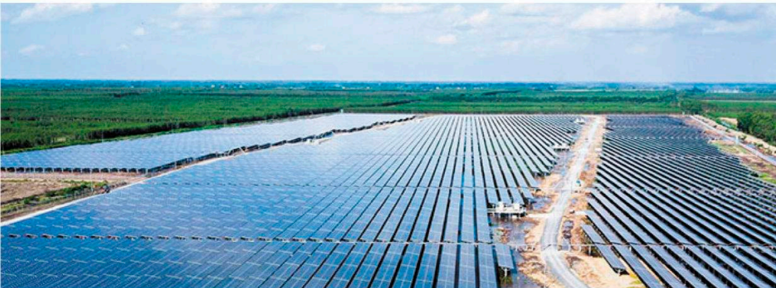
BCC-CME Long An 1 Solar Power Plant
