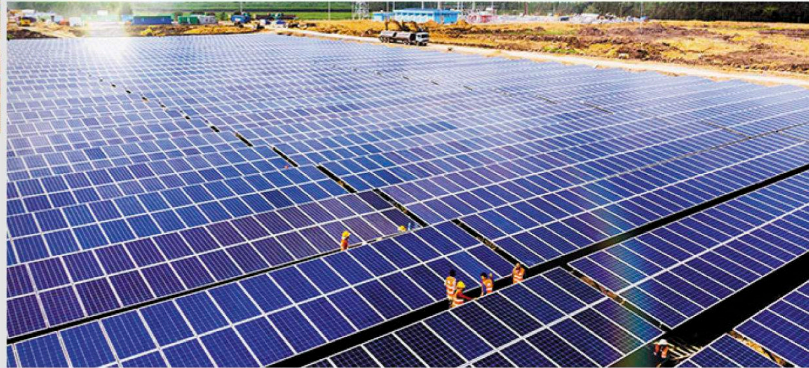
BCG-CME Long An 2 solar power plant
